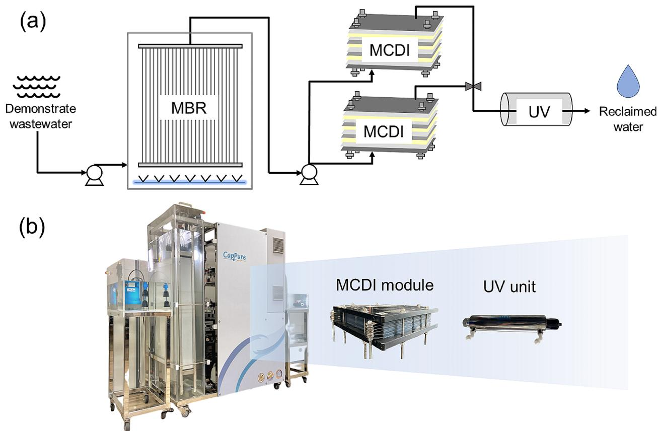
**Fig. 1** (a) Schematic diagram of the pilot-scale integrated system, (b) On-site photos of the integrated water treatment system used in field
